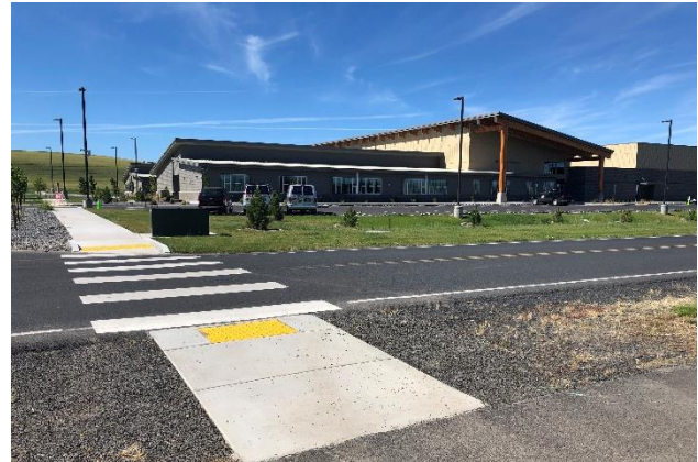
Facing south from Timine Way Trail on campus, new curb ramps and crosswalks provide safe, comfortable crossings for students.
