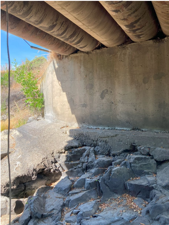
Photo 4. Dewatered dam and bridge footer left bank, Birch Creek Peterson Trust Dam.
