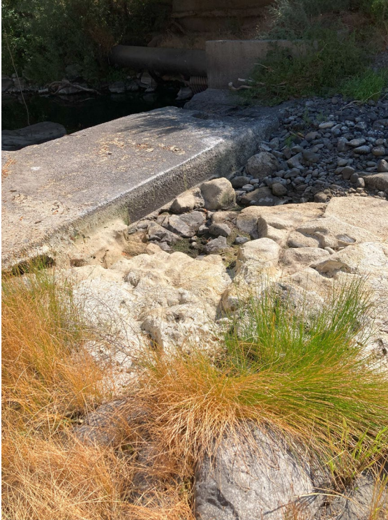
Photo 5. Upstream side of dam looking downstream and across to right bank, Birch Creek Peterson Trust Dam.
