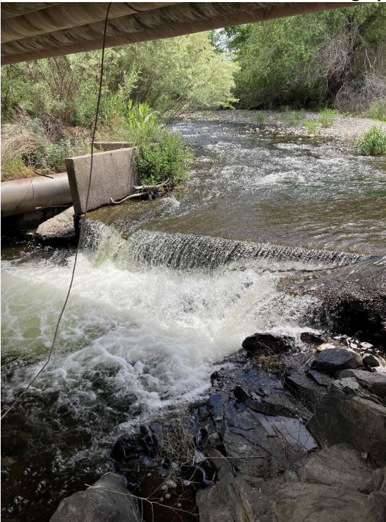
Photo 6. Downstream side of dam looking upstream, Birch Creek Peterson Trust Dam.
