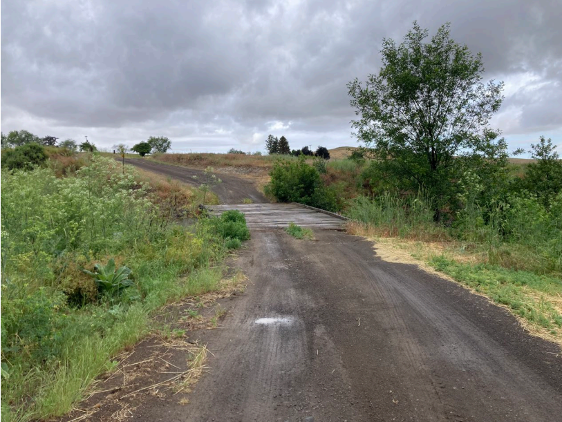
Photo 1. Access road and existing bridge, Birch Creek Peterson Trust Dam.
