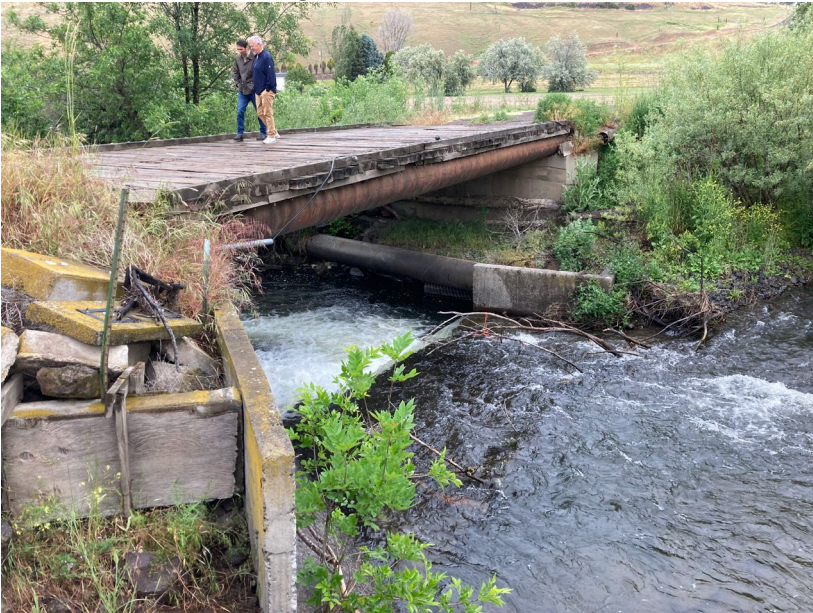
Photo 2. Dam and bridge, Birch Creek Peterson Trust Dam.
