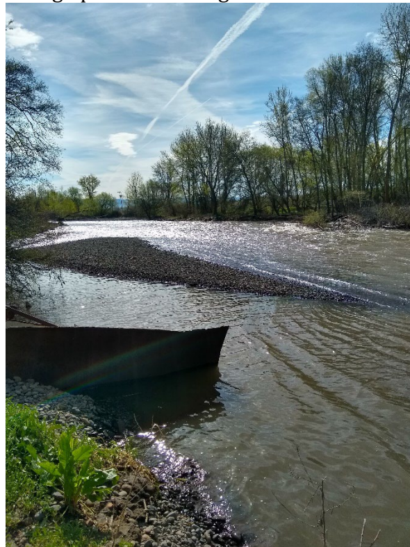
Figure 2. Looking upstream at irrigation structure near right bank
