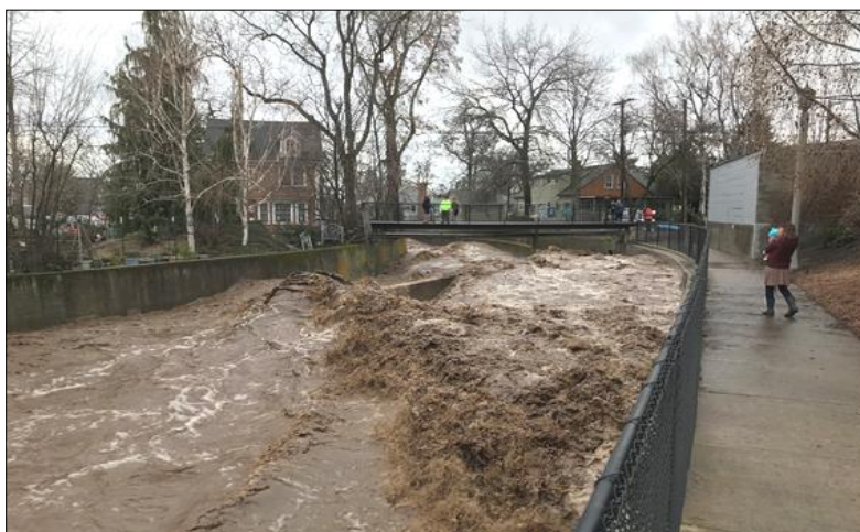
Flooding like the February 2020 event illustrates the vulnerability of infrastructure, like the Walla Walla River running through municipalities such as the City of Walla Walla pictured here.
