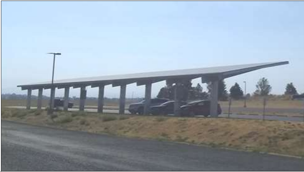
Passive energy strategies like PV shading for parking facilities. This one at TCI (pictured) provides electricity generation and reduces heat island impacts.
