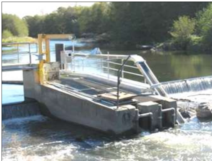
Fisheries support infrastructure like hatcheries, rearing ponds, and fish ladders could be excellent locations to co-locate microhydro generating opportunities due to their essential proximity to stream flows.
