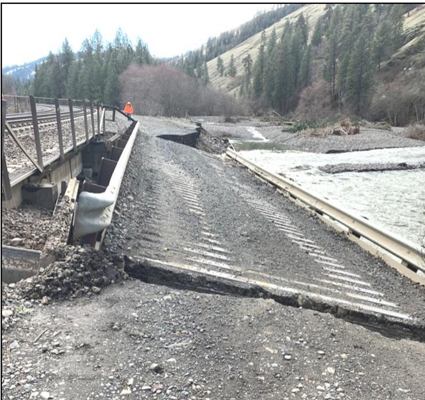
Damage to essential infrastructure from flooding, like to this railroad access bridge increases disaster recovery costs. Tribal Nations and local governments can reduce future costs by considering climate projections in current program and infrastructure development.
