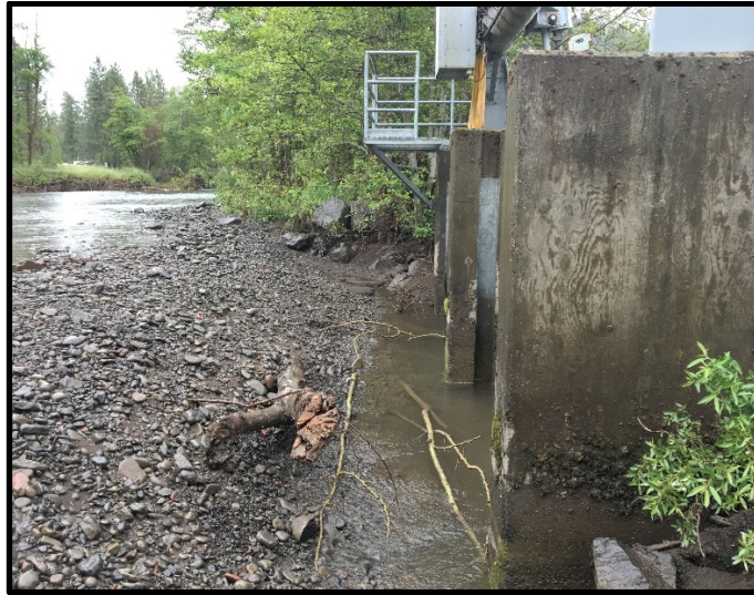
Imeqes intake structure – river elevation variance / post high water event May 2020
