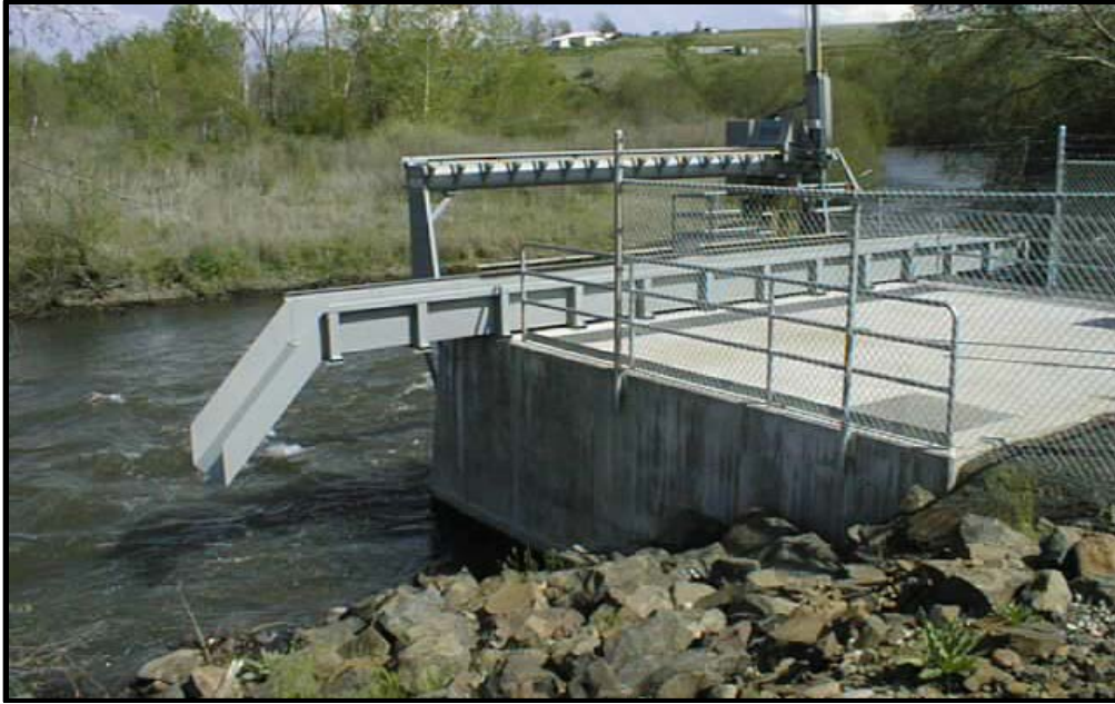
The Pendleton acclimation facility water inlet structure and associated channel that keeps sediment from inundating the inlet.
