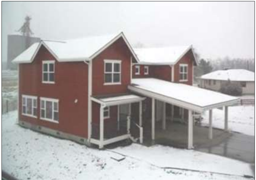
Recent Tribal housing developments like Huckleberry Court (pictured) have been built to include energy efficiency measures that can reduce energy demands and improve standard of living.
