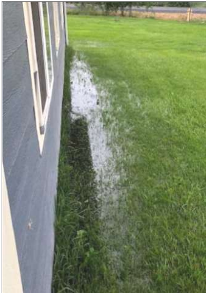
Mission area housing has experienced inundation from rising groundwaters, also known as a spring, which is located in the floodplain of nearby Mission Creek.
