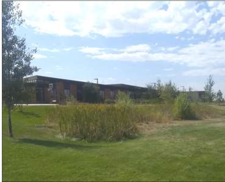
Greenspaces and other permeable surfaces like the engineered wetlands outside the Yellowhawk Tribal Health Center (pictured) help stormwater be infiltrated rather than pooling.
