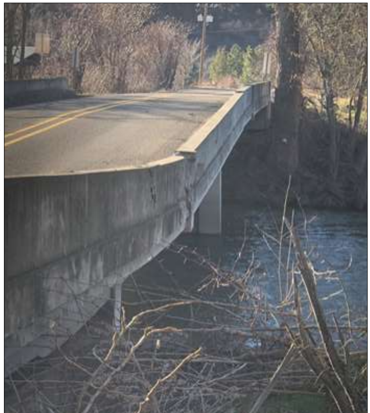
Thornhollow Bridge on the Umatilla Indian Reservation was damaged by the February 2020 flooding. Note the buckled concrete in the bridge center.
