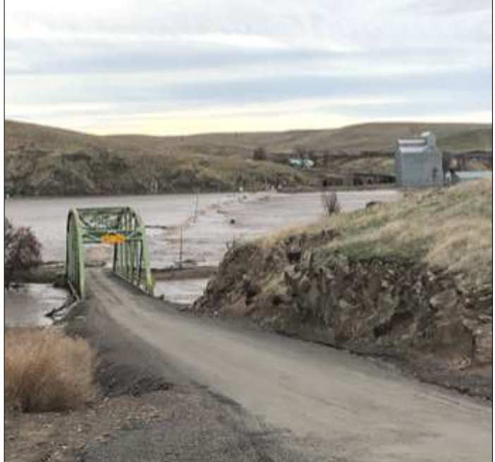
Previous flooding events like the one on the Umatilla River in Feb 2020 have revealed where regional infrastructure is vulnerable to future disaster events.
