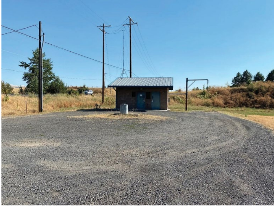
Fig.3 Well 4 Site 46443 Mission Road Pendleton, OR 97801
