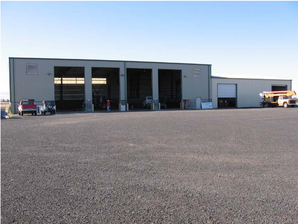
Figure 3.1 Tribal Environmental Recovery Facility (TERF)
