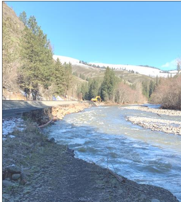
River-adjacent infrastructure, such as the Union Pacific Railroad line along Meacham Creek (pictured left), is threatened by flooding and also impedes floodplain reconnection.
