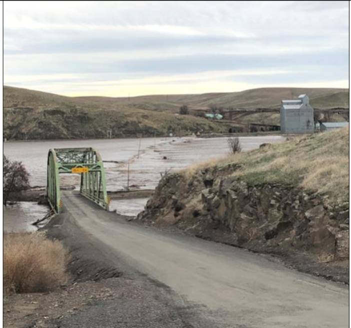
Previous flooding events like the one on the Umatilla River in Feb 2020 have revealed where regional infrastructure is vulnerable to future disaster events.
