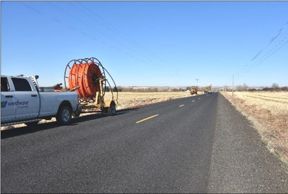
Broadband Internet cable is installed across much of the Mission and Tutuilla areas of the UIR, and is usually laid concurrently along established roads.
