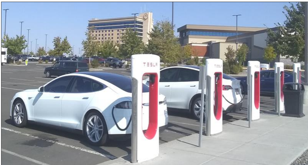
Electrification of tasks and services could facilitate a shift to renewable energy, though investment in infrastructure is necessary to making this successful. Electric vehicle (EV) charging stations like the one at Wildhorse Resort and Casino (pictured) expand the capacity of EV feasibility, as “range anxiety” for these vehicles is cited as a large barrier to their wide-spread implementation.
