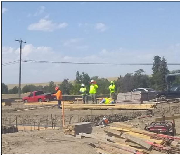
Construction workers take a break from work on the new Nixyaawii apartment buildings under extreme heat which will become more frequent.
