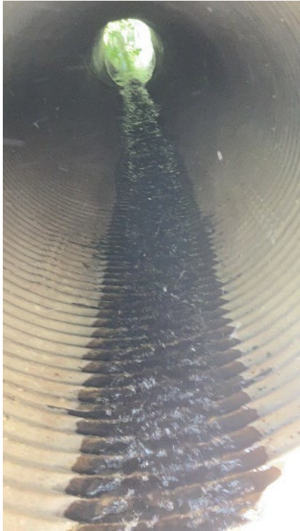
Photo 4. Moonshine Creek culvert looking downstream, August 7, 2025.
