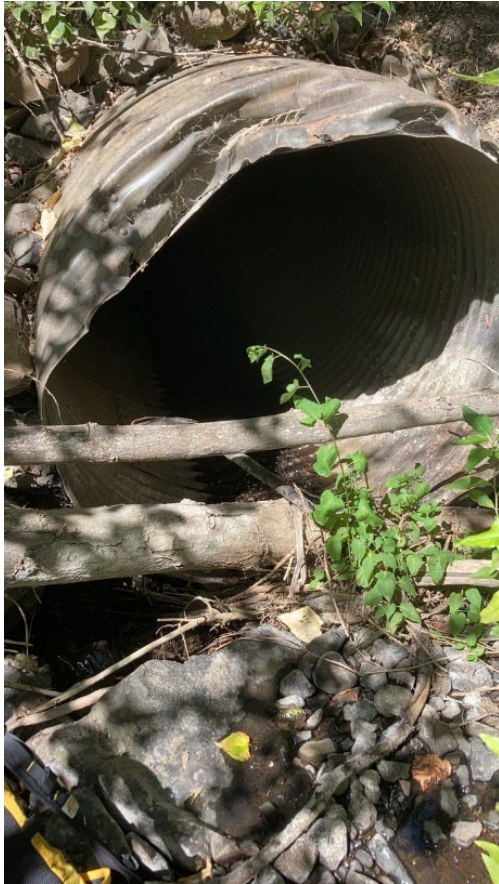
Photo 5. Moonshine Creek culvert upstream side, August 7, 2025.
