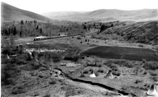
RAILROAD, UMATILLA INDIAN RESERVATION (PHOTO COURTESY TCI)
