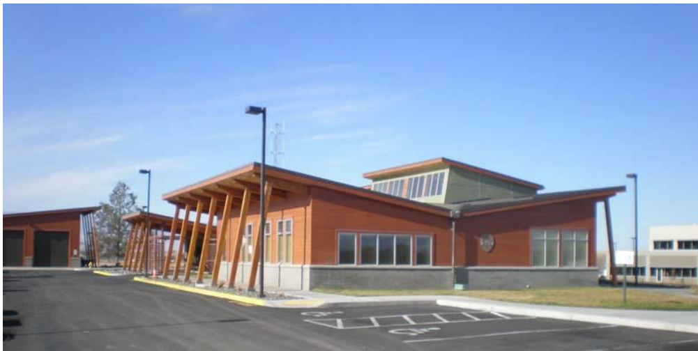
PUBLIC SAFETY BUILDING (CTUIR PHOTO)
