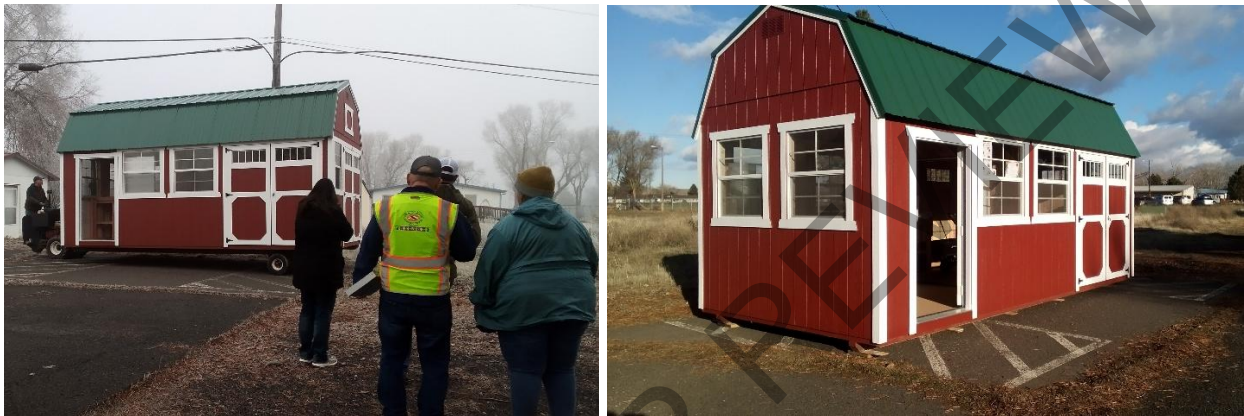
Images [67 and 68]: Project team members and staff from CTUIR Tribal Planning Office are present for the installation of the project shed in January 2025.
