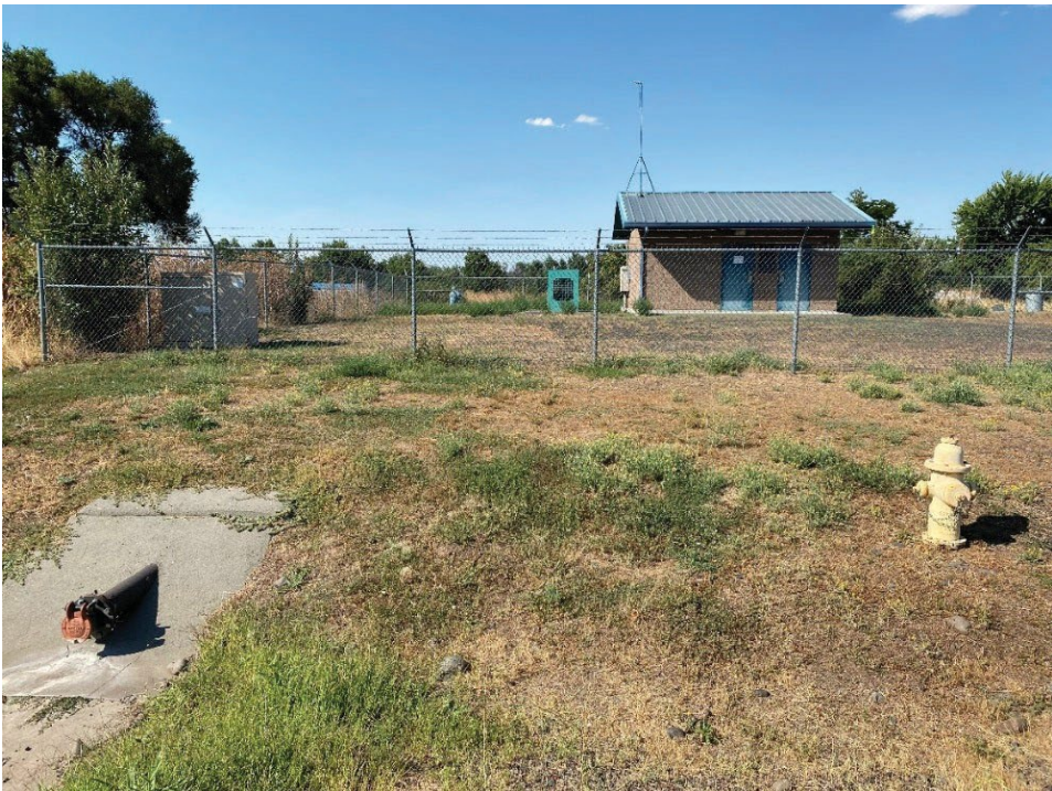
Fig.2 Well 3 Site 47563 Short Mile Road Pendleton, OR 97801
