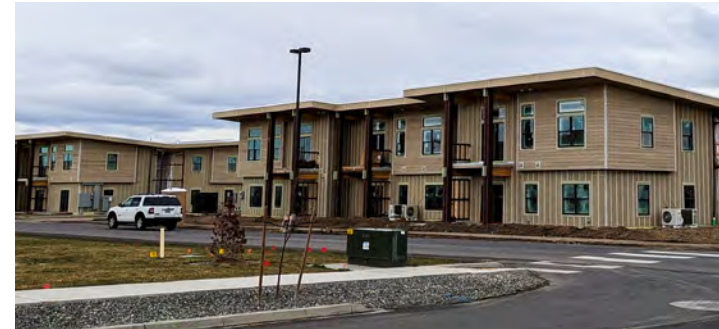
Timine Way North Apartments
