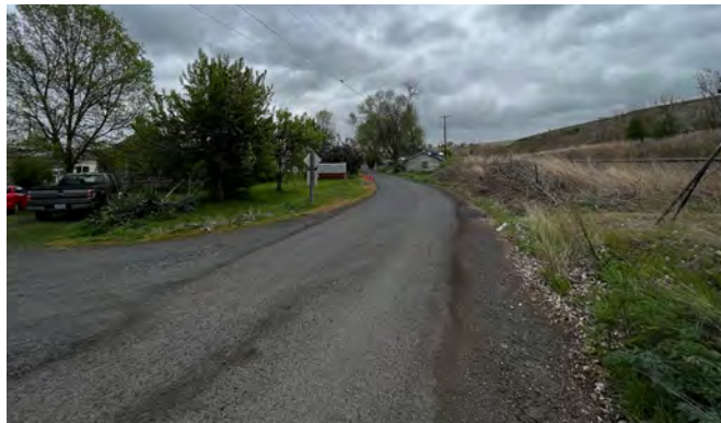
Mytinger Lane near the mobile home park before road veers north
