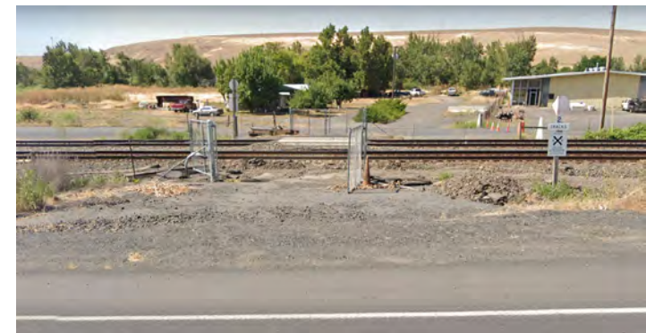
3 Inactive railroad crossing at McKay Lane Source: Google Earth
