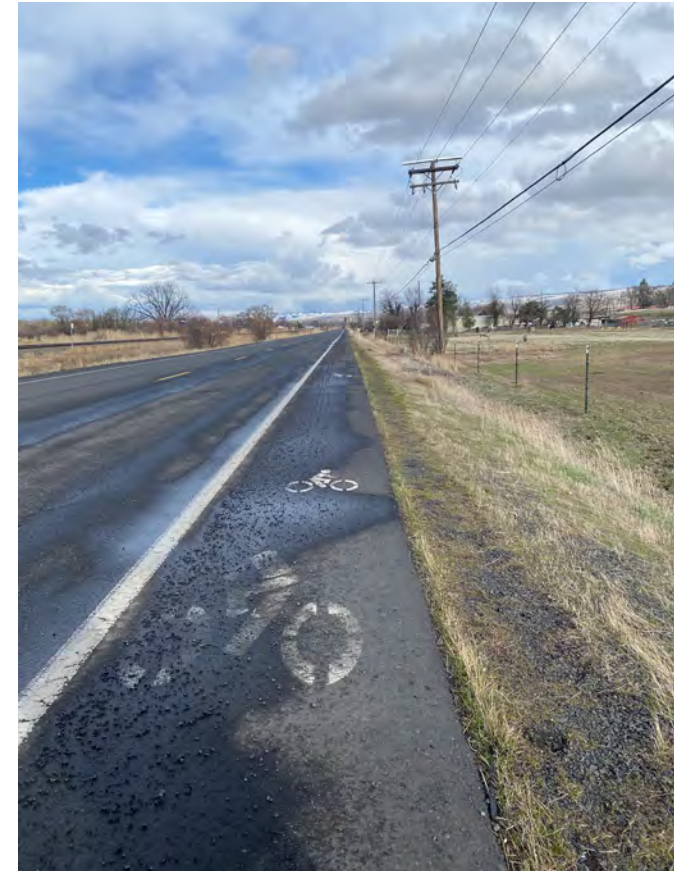
Marked shoulder bikeway along Mission Road
