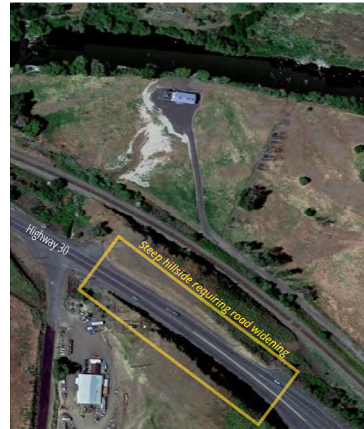
Figure 22. Highway 30 surrounded by steep hillside
