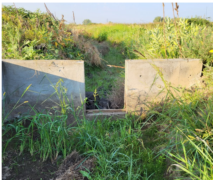
Figure 4. Example of irrigation canal cross regulator (removable boards not shown), to be installed at CRD1 and SW02b (Task 2)
