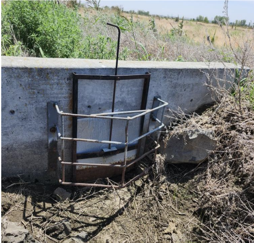
Figure 1. Example of water control stop gate in closed position (at water control structure M05).
