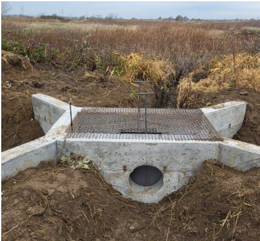
Figure 6. Example of headgate structure, to be installed at M03b (Task 3)
