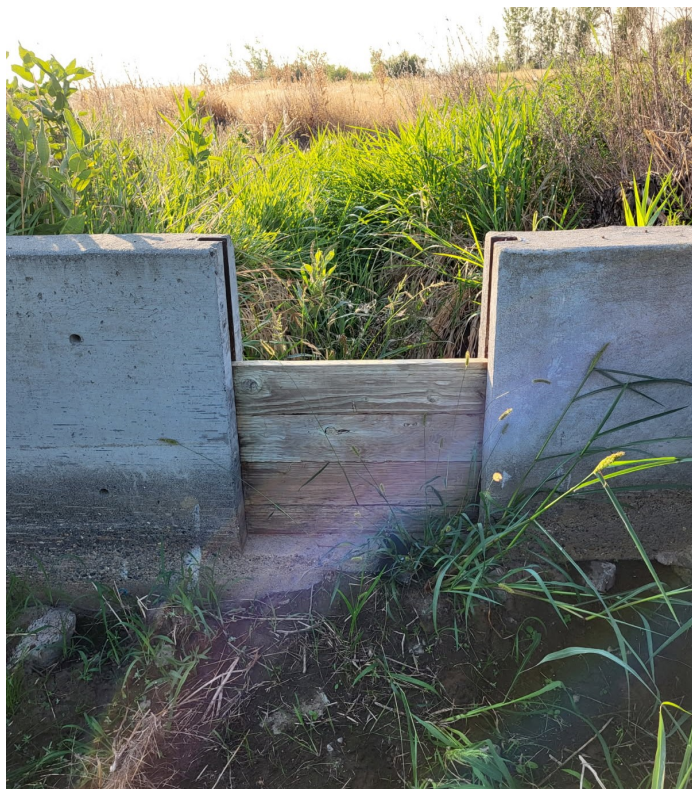
Figure 3. Example of irrigation canal cross regulator with removable boards, to be installed at CRD1 and SW02b (Task 2)
