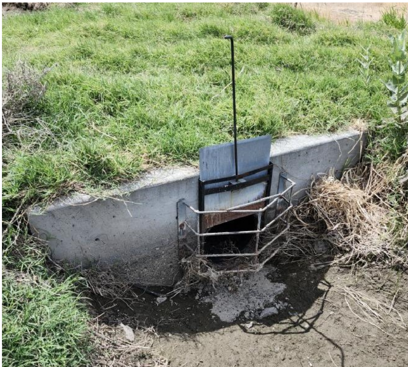
Figure 2. Example of water control stop gate in open position (at water control structure SM01)
