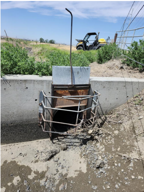
Figure 8. Water control stop gate and “spillway”, both to be replaced, at M03b (Tasks 1 and 4)
