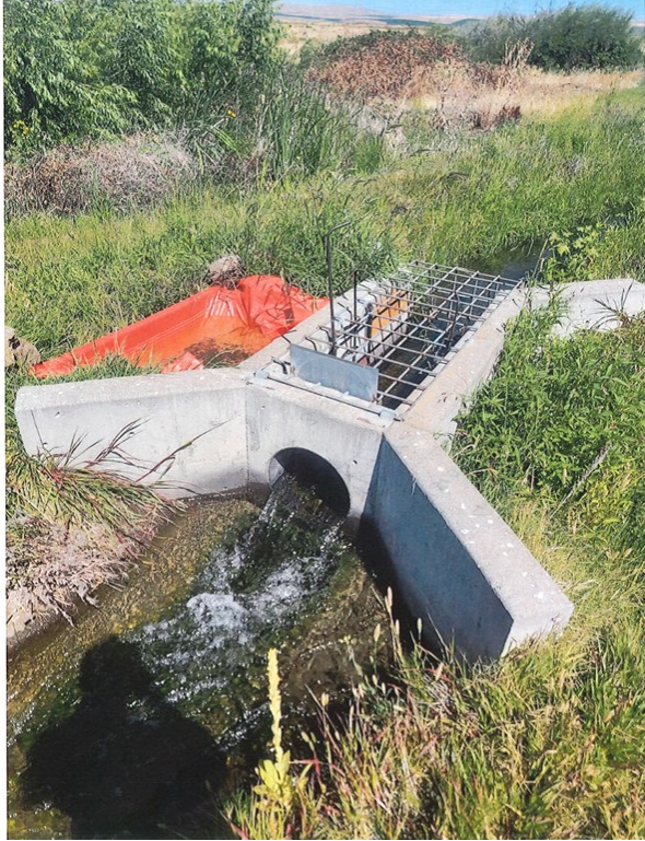
Figure 7. Example of headgate structure to be installed at M03b (Task 3)
