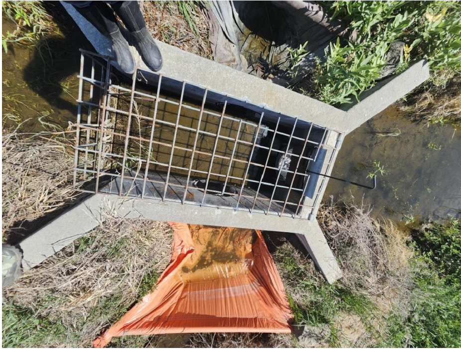
Figure 5. Example of headgate structure, to be installed at M03b (Task 3)
