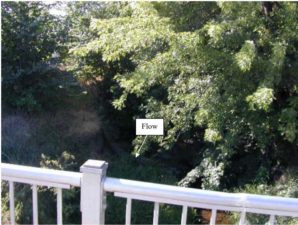
Photo No. 45: View looks upstream (east) at Tutuilla Creek from bridge on Hailey Ave.
