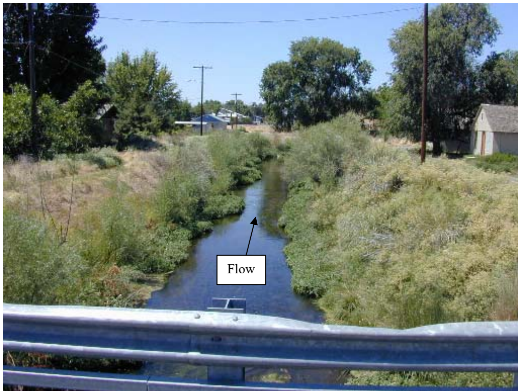
Photo No. 66: View looks downstream (west) from Dunne St. bridge.
