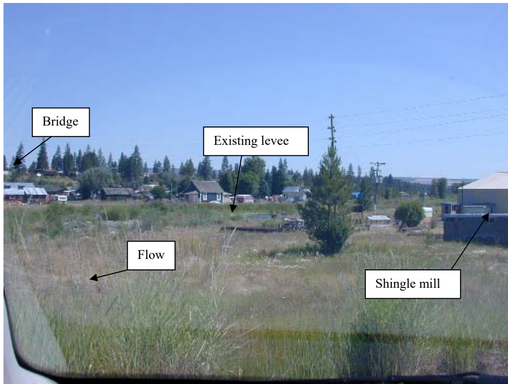
Photo No. 74: View looks east at Camas Creek (on south edge of town). Taken from south end of bridge on Soap Hill Road.
