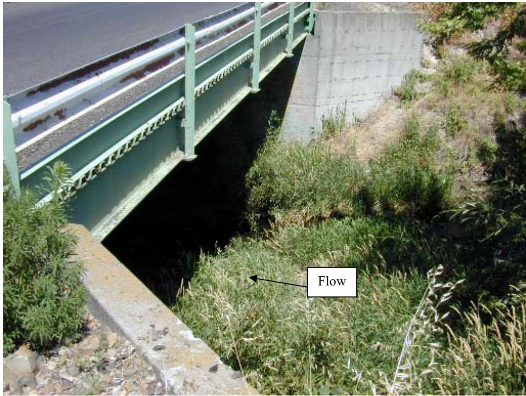
Photo No. 17: View looks at upstream face of bridge.
