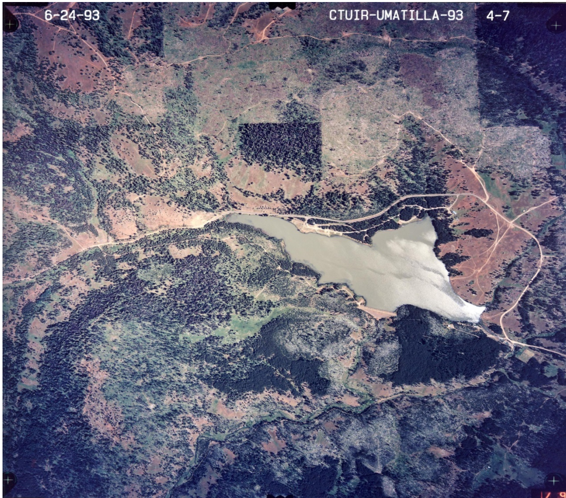
Indian Lake Dam
