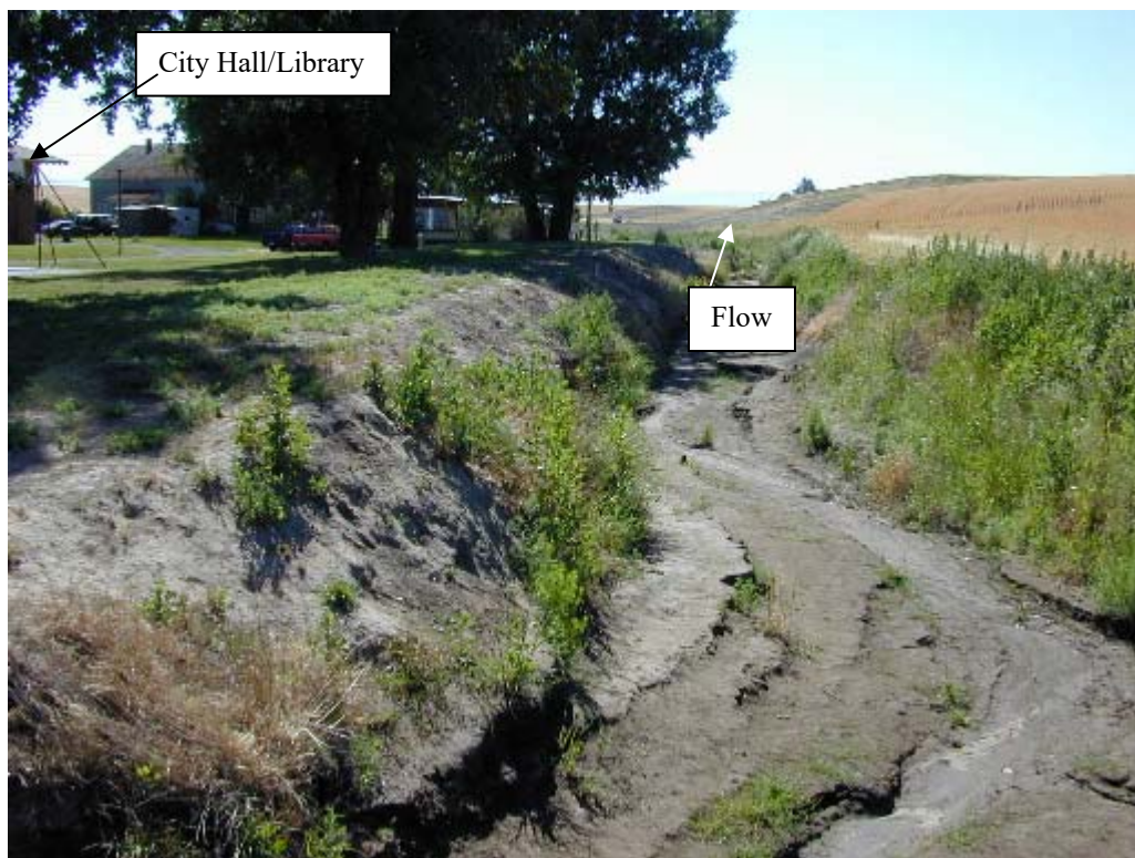
Photo No. 34: View looks southeast at Greasewood Creek, looking downstream.
