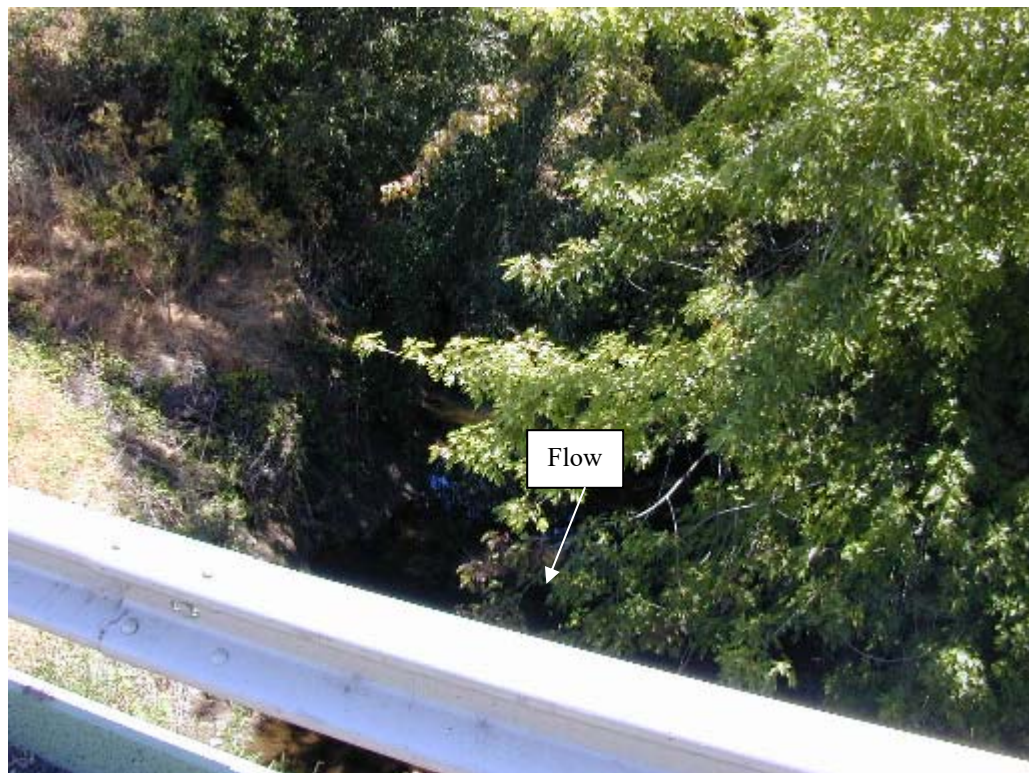
Photo No. 16: View looks upstream (north) at combined Waterman Creek/Wildhorse Creek south of town.
