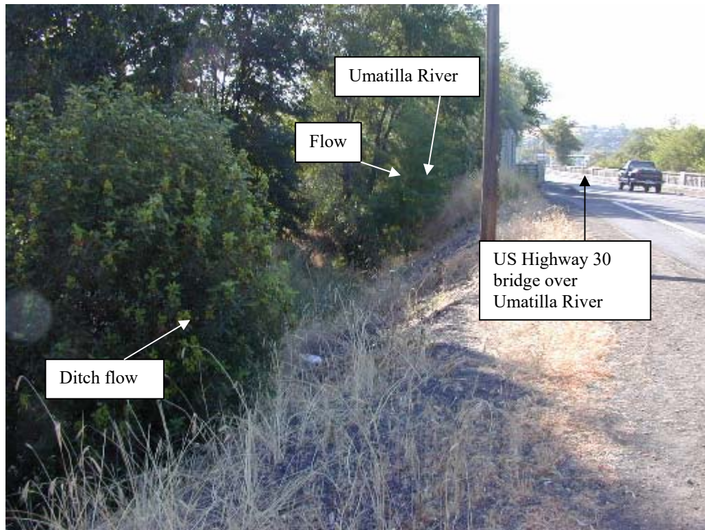
Photo No. 43: View looks east at Nelson Creek ditch to Umatilla River.
