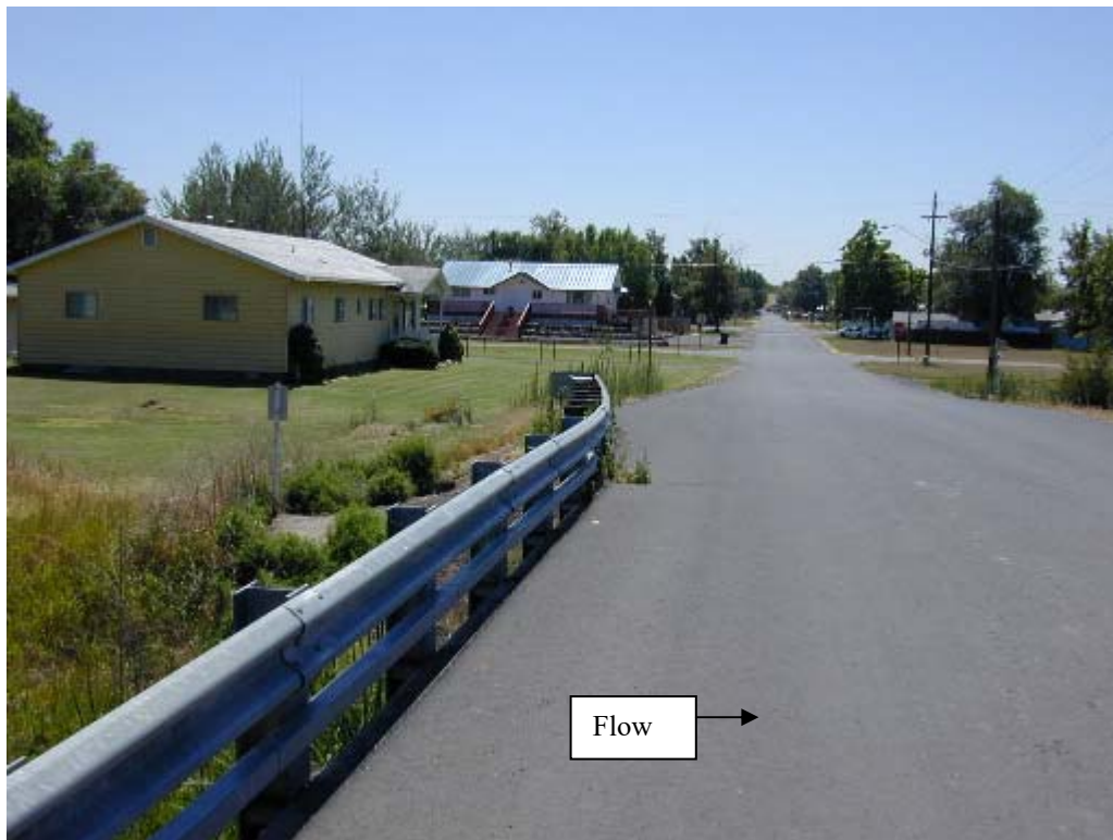
Photo No. 65: View looks south from bridge on Dunne St.
