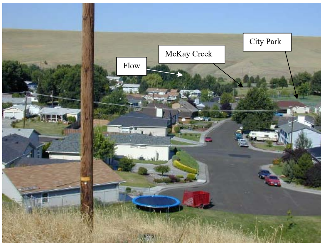
Photo No. 53: View looks southwest at Montee Addition where flooding has occurred in the recent past.
