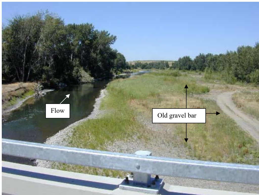
Photo No. 19: View looks downstream (north) at gravel bar downstream from bridge site.
